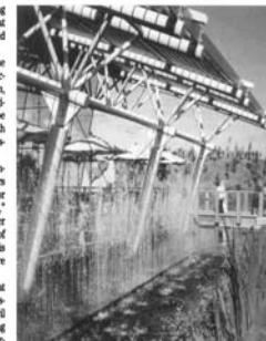
Landmark projects such as the M40 Wheatley service station demonstrate that sustainable development is now “absolutely central” to civil engineering.
