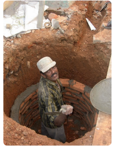
Leach pit under construction
