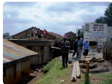
Bio-latrine under construction
