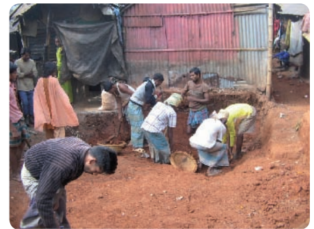
Excavating 1st Infrastructure in Slums
