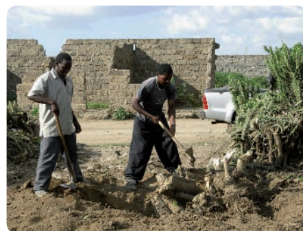
Preparing the site in Karagita for water treatment tanks
